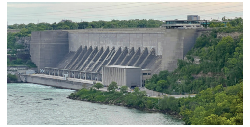
The Robert Moses Niagara Hydroelectric Power Station
